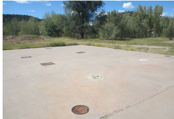
PHOTOGRAPH No. 10 View of UST area
